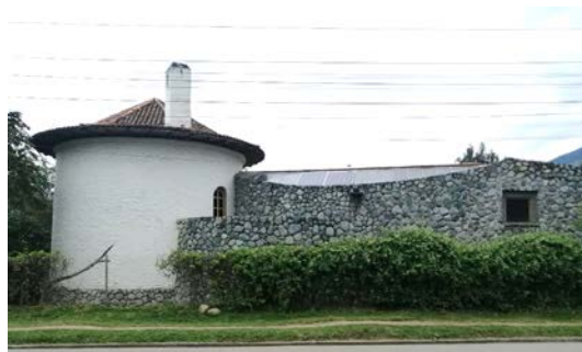
Fig. 5. Side view of the house with the photovoltaic system under study.
