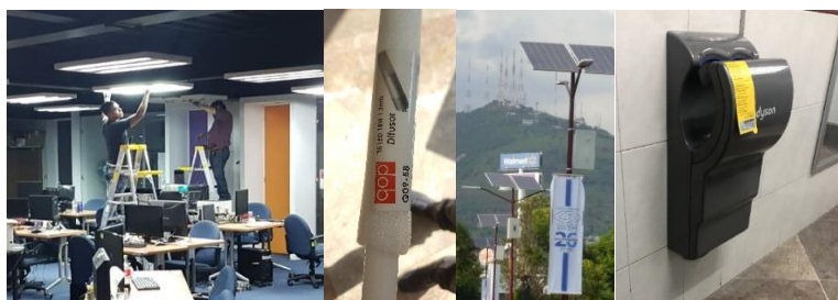
Fig. 6. Replacement of luminaires, PV luminaires and low consumption hand drier.
