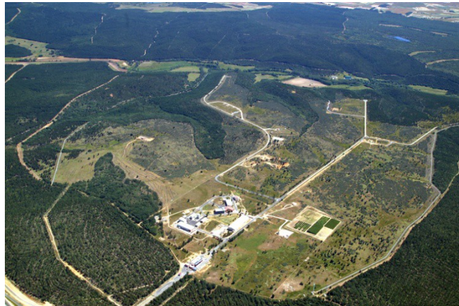
Fig. 1. Aerial image of CEDER. The center is located on 640 ha of land. Courtesy of CEDER.
