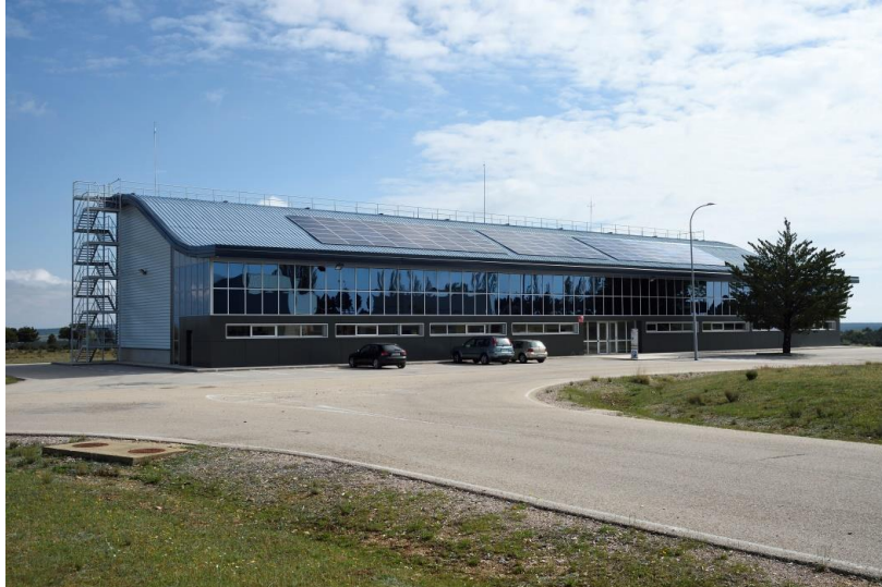
Fig. 1. Photovoltaic system in the rooftop of the offices of CEDER in Lubia (Soria, Spain). Image courtesy of: CEDER.
